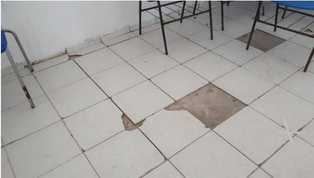
**FOTO 13:** VISTA DE PISO CERÂMICO A REVITALIZAR P/ KORODUR.
