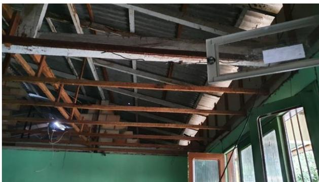
**FOTO 03:** DETALHE DA COBERTURA TODA DETERIORADA, INCLUSIVE FORRO E ELÉTRICA.
